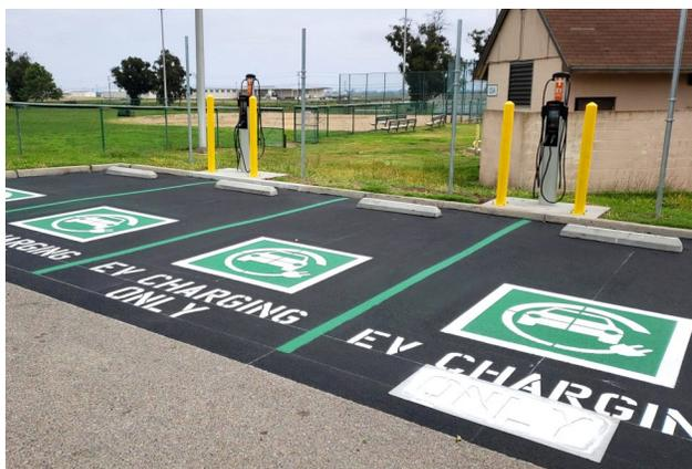
*Picture of two Level 2 charging stations for Private Owned Vehicles at the installation's Navy Exchange.*
