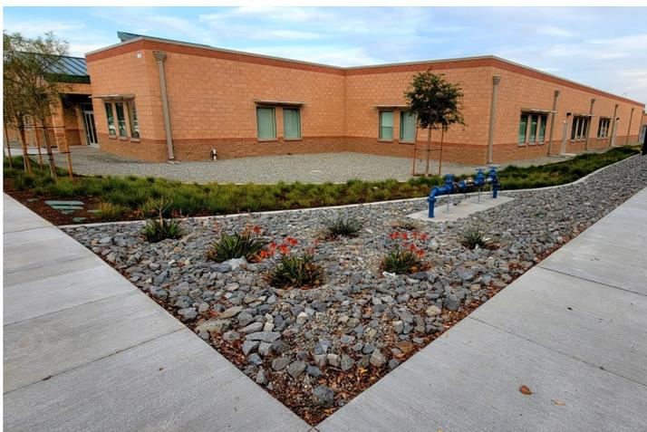
*Erosion control at the Seal Beach Reserve Center. The installation installed multiple retention basins and LIDs to ensure building and surface runoff is captured before draining into adjacent channels leading to the Anaheim Bay.*
